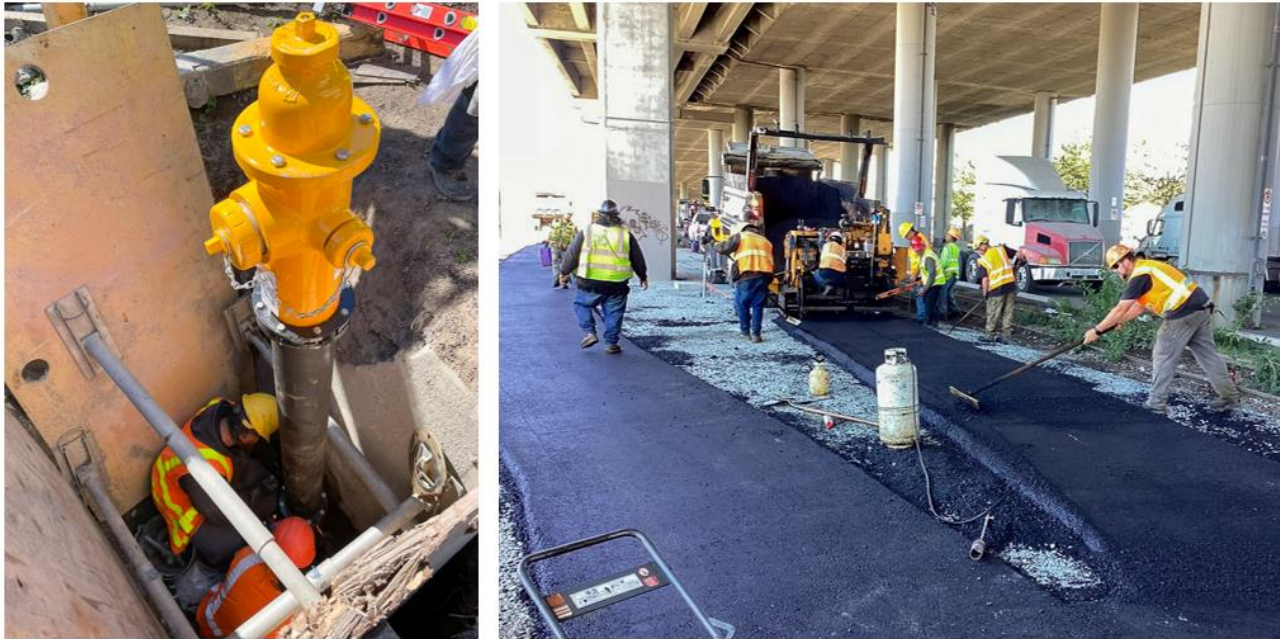
Installing a fire hydrant (left) and laying asphalt for new protected bike lanes (right) along East Marginal Way.
