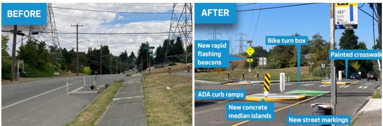
Before (left) and after (right) improvements at 51st Ave S and S Gazelle St.
